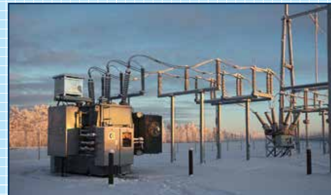
As electrical power substations become more complex, cybersecurity of substations must become a priority. (Photo courtesy of U.S. Corps of Engineers, Clear Air Force Station, Alaska)
