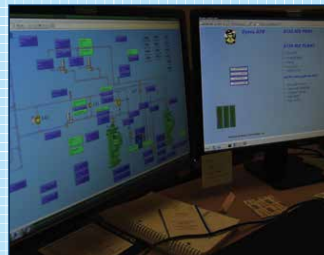
Airmen and contractors use an energy management control system to remotely monitor air-conditioning systems on Dyess Air Force Base, Texas. (U.S. Air Force photo/Senior Airman Alexander Guerrero)
