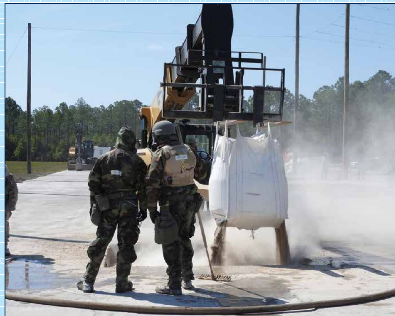
Below: Airmen practice rapid airfield crater repair techniques while testing new protective lightweight clothing for AFCEC's Civil Engineer Laboratory on Tyndall Air Force Base, Florida. (U.S. Air Force photo/Mekka Parish)
