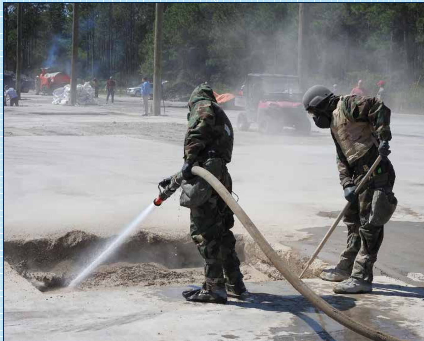
Airmen practice airfield damage repair techniques while testing lightweight protective suits. (U.S. Air Force photo/Mekka Parish)
