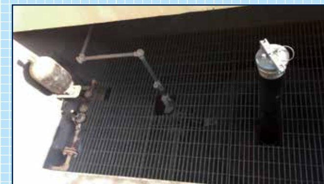
Top: Vaulted above-ground storage units allow for plug-and-play fuel operations for mission enhancements and reduced downtime.
